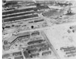
Early construction at Fort Benning--29th Infantry Barracks, circa 1924. ( U.S. Army Collection, National Archives )
